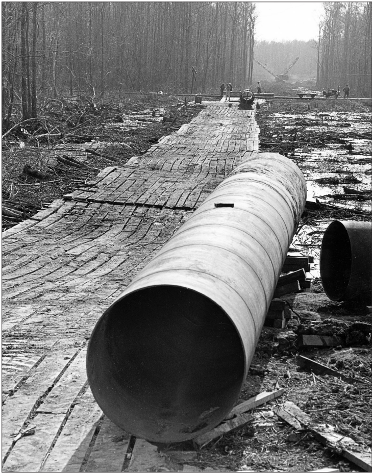
1968: A view of the Capline System's "spread No. 1" between New Orleans, La., and Baton Rouge, La. The rainy winter of 1968 hampered construction of the pipeline. Planks such as those shown here helped workers and equipment move from place to place without sinking in the mud.
