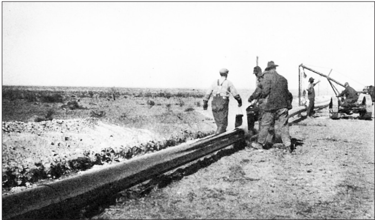
1927: Rex Martin's crew uses a 'granny rag' to coat a section of the McCamey-Cushing Pipeline with tar.
