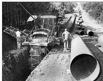
(above) 1958: A joint of a natural gas pipeline is welded aboard a lay barge on Lake Pontchartrain in Louisiana. The line ran from four wells in Lake Pontchartrain to Shell's Norco Manufacturing Complex. (right) 1967: A huge ditching machine cuts a deep path along the Capline System right-of-way.
