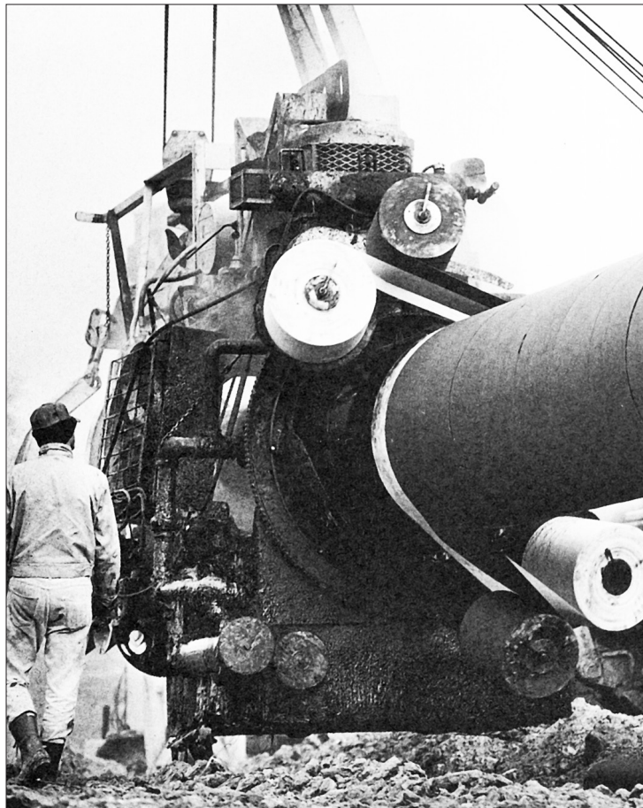
1968: A sophisticated pipeline wrapping machine quickly covers a section of the Capline Pipeline.
