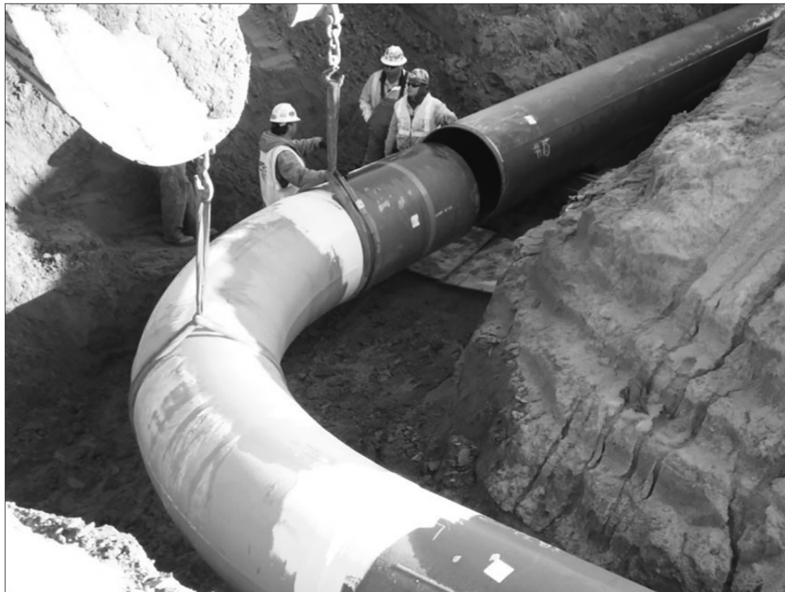
2013: Aligning a 90° bend during a re-route of the Capline pipeline to accommodate an interstate expansion in Mississippi.
