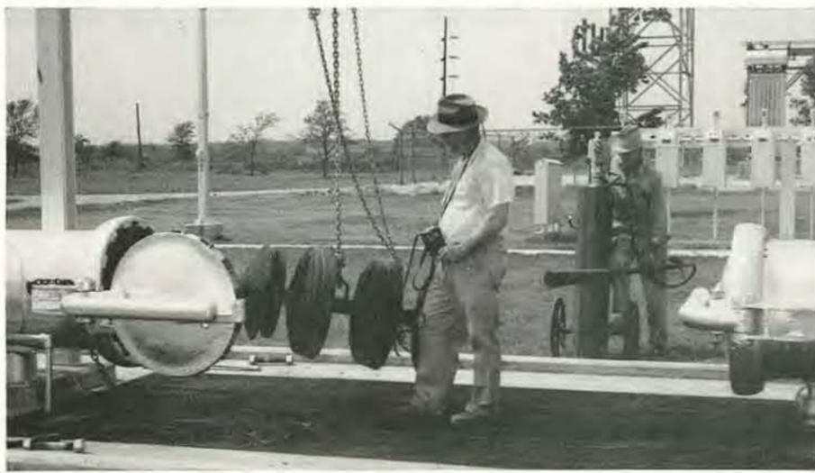
L. L. Arnold, Garfield Station assistant chief engineer, puts a plug-type cleaner into the 24-inch Rancho Pipe Line System while checking a gas detector in his right hand. The man manning the fire extinguisher is R. D. Webb, utilityman.
