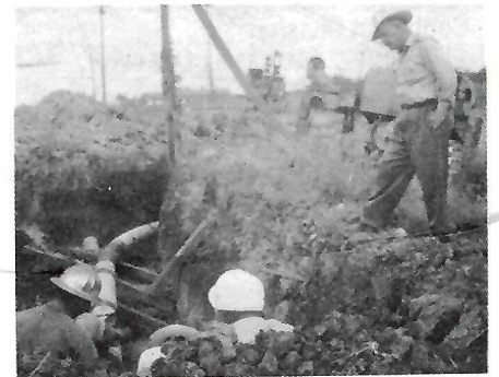
C. C. Moss, maintenance foreman at Goodrich, Tex. and inspector for the relocation project, observes the installation of the end coupling for the east end tie-in of the Shell-Sinclair line.
