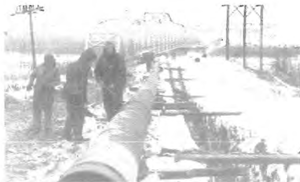
Severe winter weather challenged the working abilities of the men who were relocating the Ozark System's mainline Missouri River crossing. Despite the severe cold, little more than three months were needed to complete the job.
