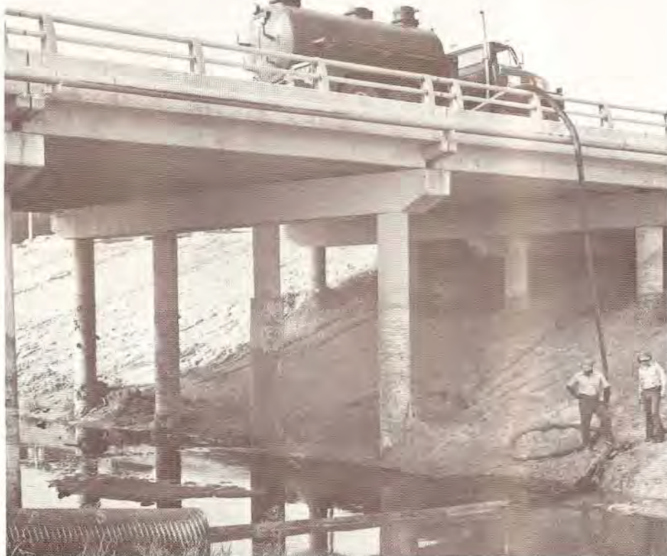
A vacuum truck sucks oil from Brays Bayou near the boom containing the crude.
