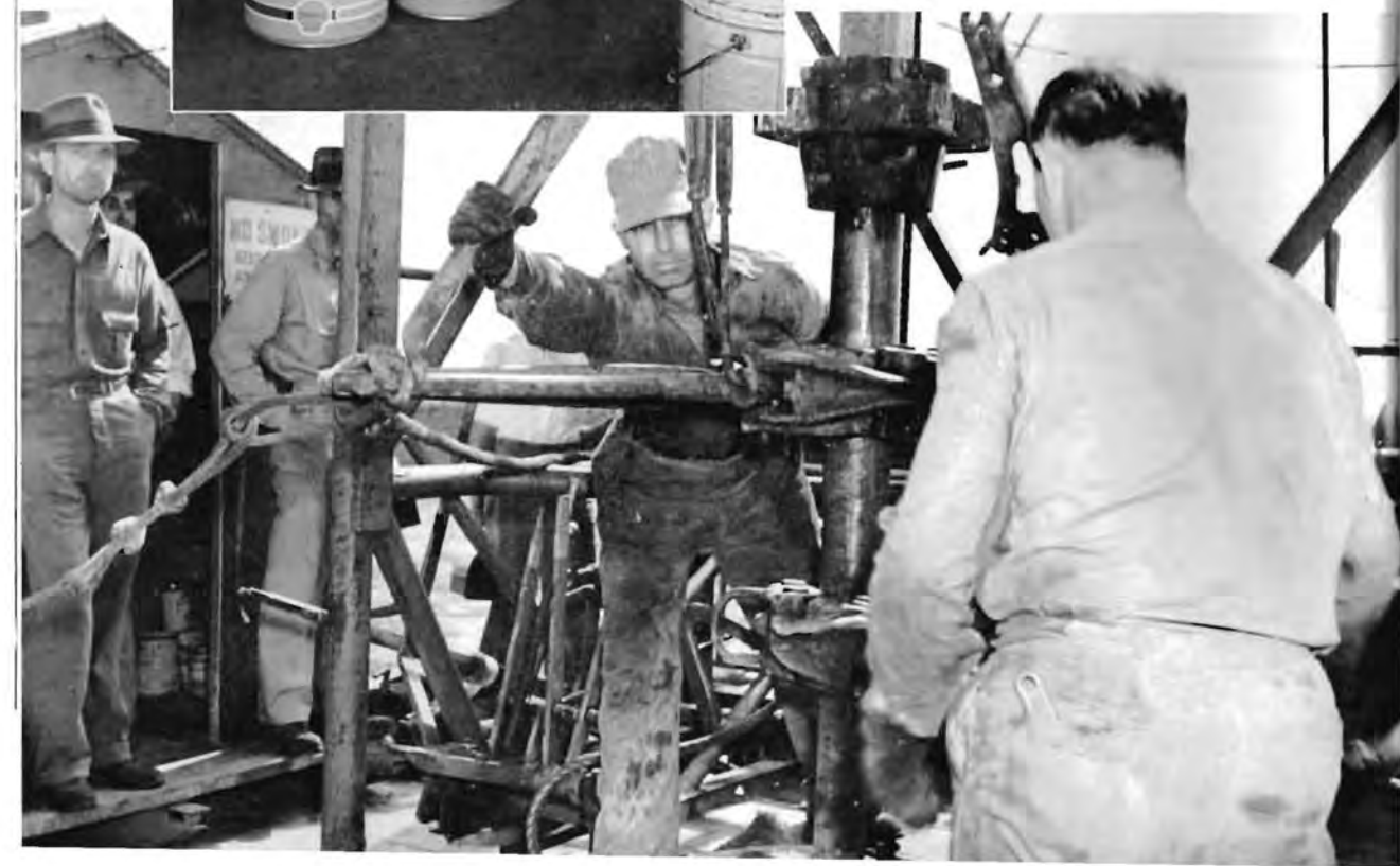
(Below) Crew setting up Kelly joint on portable drilling plant unit at M. Dumler No. 12, Trapp pool, Russell County, Kansas.
