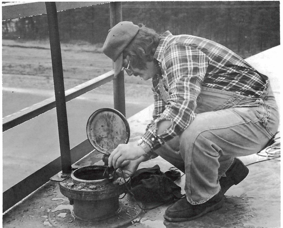
Mike periodically checks the temperature inside the storage tanks.
