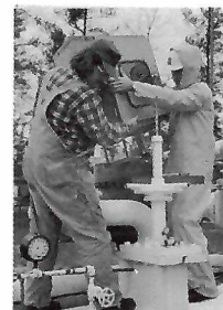
Mike Vinitski and Caroll Hughlett place the protective cover on the meter after finishing repair work on a dismantled meter skid at the Lewiston Station in northern Michigan.
