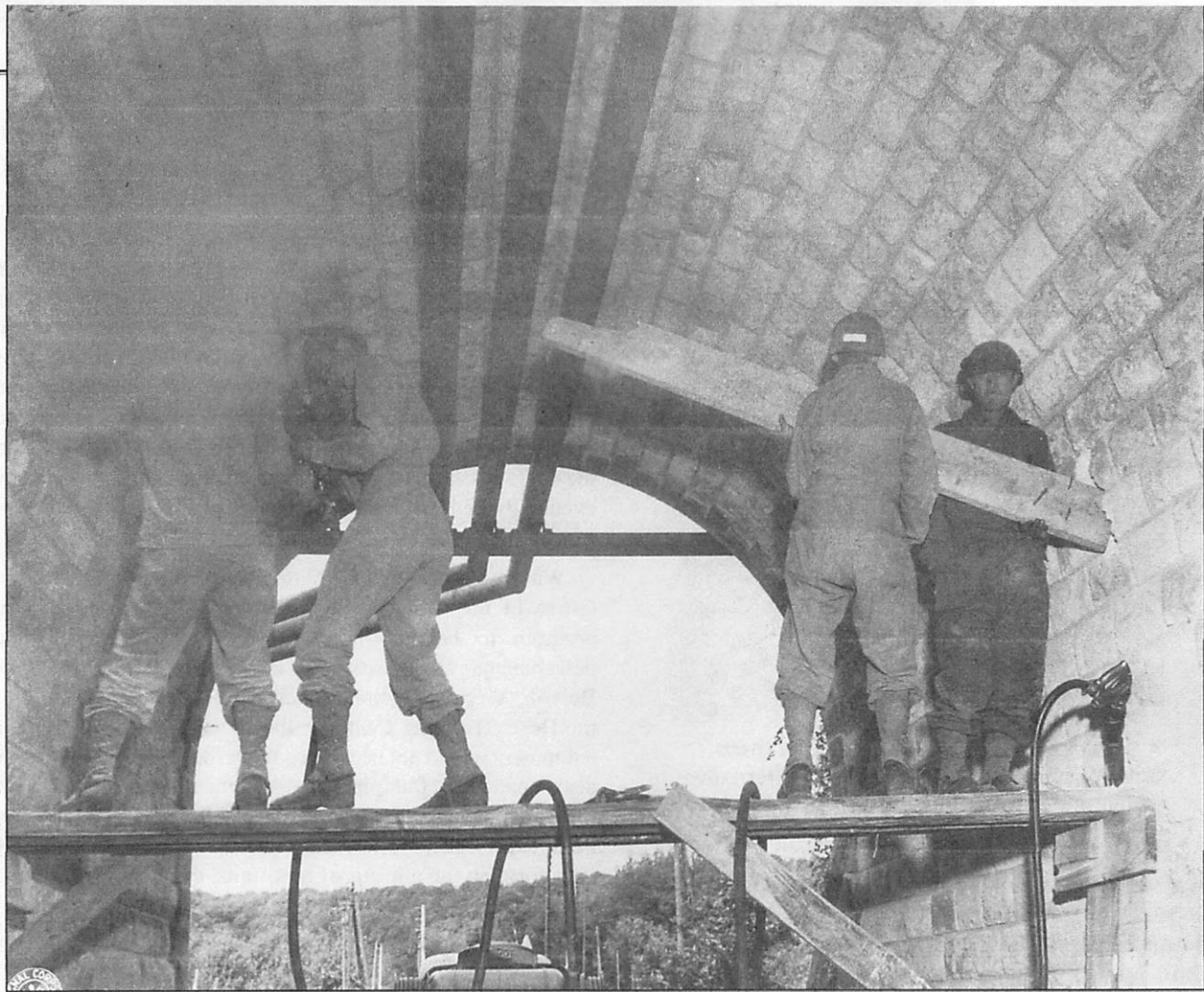
American engineers work on a stone bridge to add support for sections of a petroleum pipeline. France 1944
