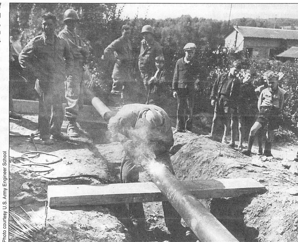
A Soldier welds sections of 8-inch pipe that will bring fuel to Allied aircraft, armor, and motor transport in France. September 1944
